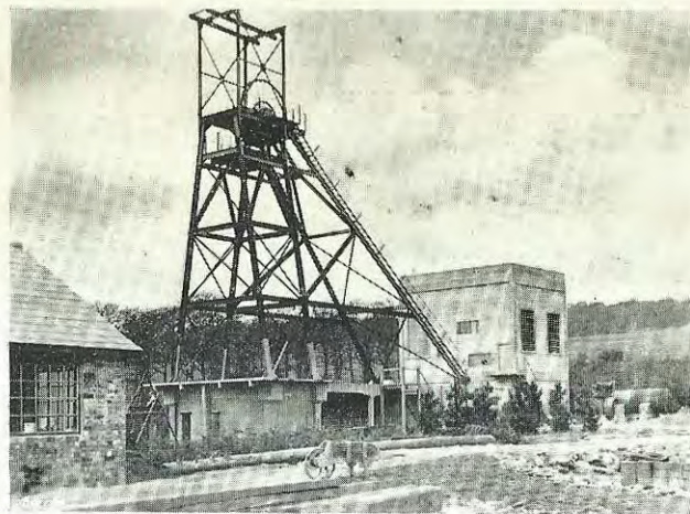
HENRY CRAWSHAY & CO.'s NORTHERN UNITED COLLIERY, showing new Head Stocks before sinking commenced
