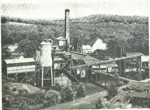
CANNOP COLLIERY, showing new Dry Cleaning Plant in operation
